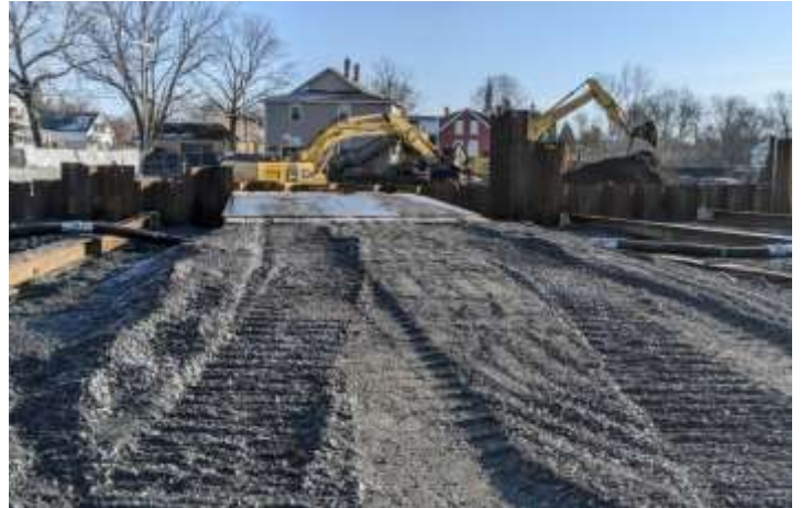
Access Over Temporary Bypass Channel
