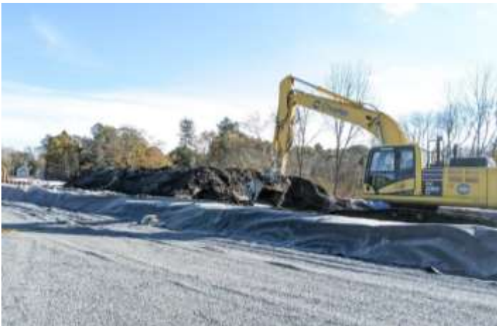
Dewatering Excavated Soils
