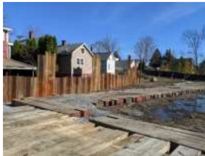
Support Mats Positioned for Accessing Excavation Area
