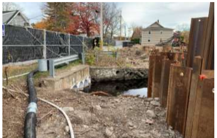
Mire Brook at Commonwealth Ave with Excavation Sheet Piling
